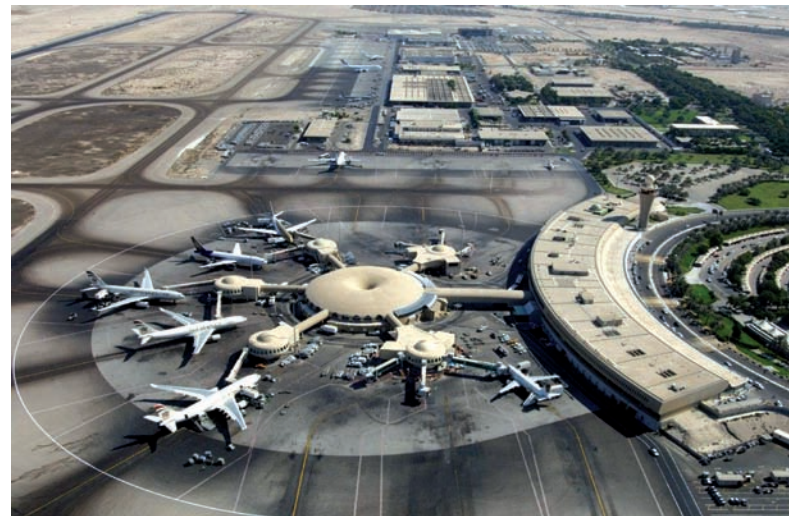
Abu Dhabi International Airport
